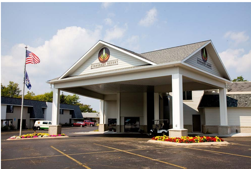
View at the main entrance as you arrive at Evergreen Resort in Cadillac.
